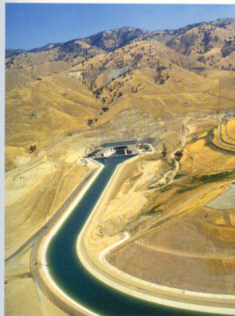
Plate 58. The A.D. Edmonston Pumping Plant, which lifts SWP water almost 2,000 feet over the Tehachapi Mountains.
