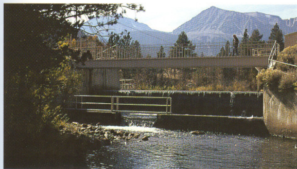
Plate 71. Lee Vining Creek at the point where water is diverted from the Mono Lake tributary into the Los Angeles Aqueduct.
