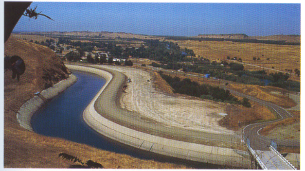
Plate 67. The Friant-Kern Canal, heading southward below Friant Dam and leaving very little water for the San Joaquin River, seen in the distance.
